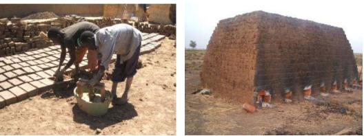
Fig. 3 - Manual brick forming.
